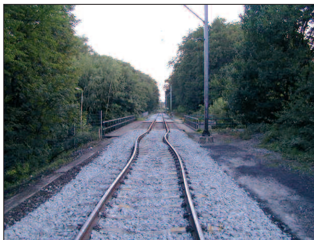
Fig. 2: Track buckling
